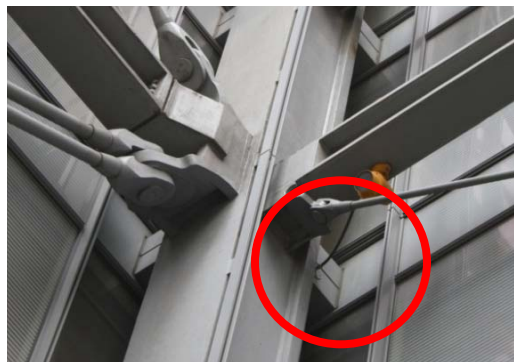
FIGURE 2- 'Dog-leg' penetrating building envelope
